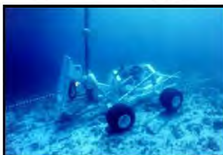
Power cable installation using Hydroplow
