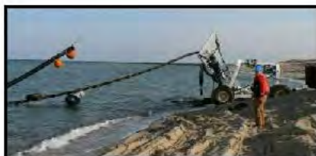
Power cable installation using Hydroplow
