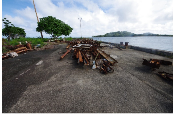
Main Wharf Area
