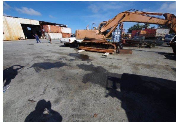
Oil leak from machinery at Yap Port
