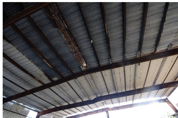
Roof of Port Warehouse
