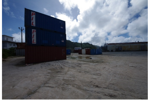
Water pooling in Container Yard
