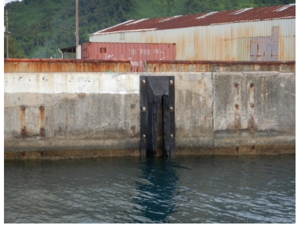
Damaged fender
