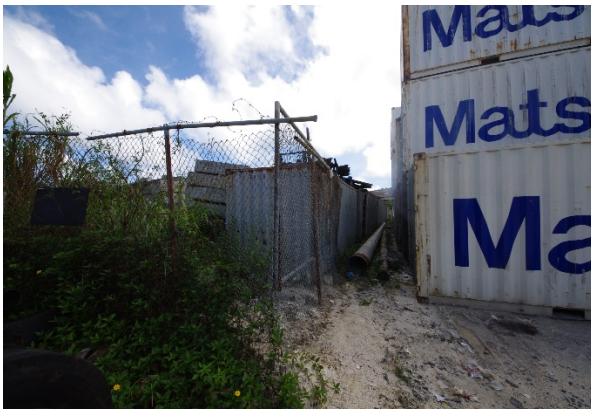
Containers being used as a fence
