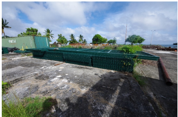
New Fencing Infrastructure awaiting installation
