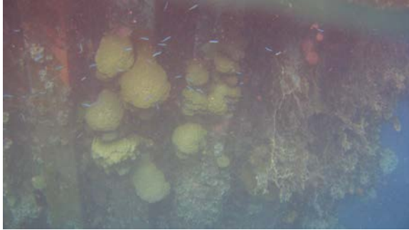
Sheet Piling at Tonoas Port
