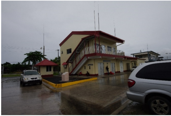
Port Security Office
