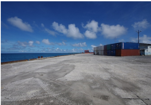
Main Berth Wharf frontage
