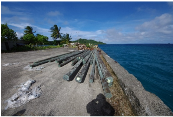
New Light Poles awaiting installation
