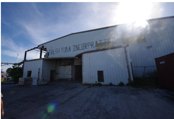
Derelict Fresh Tuna Incorporation Building
