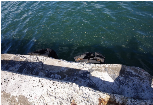
Damaged fender
